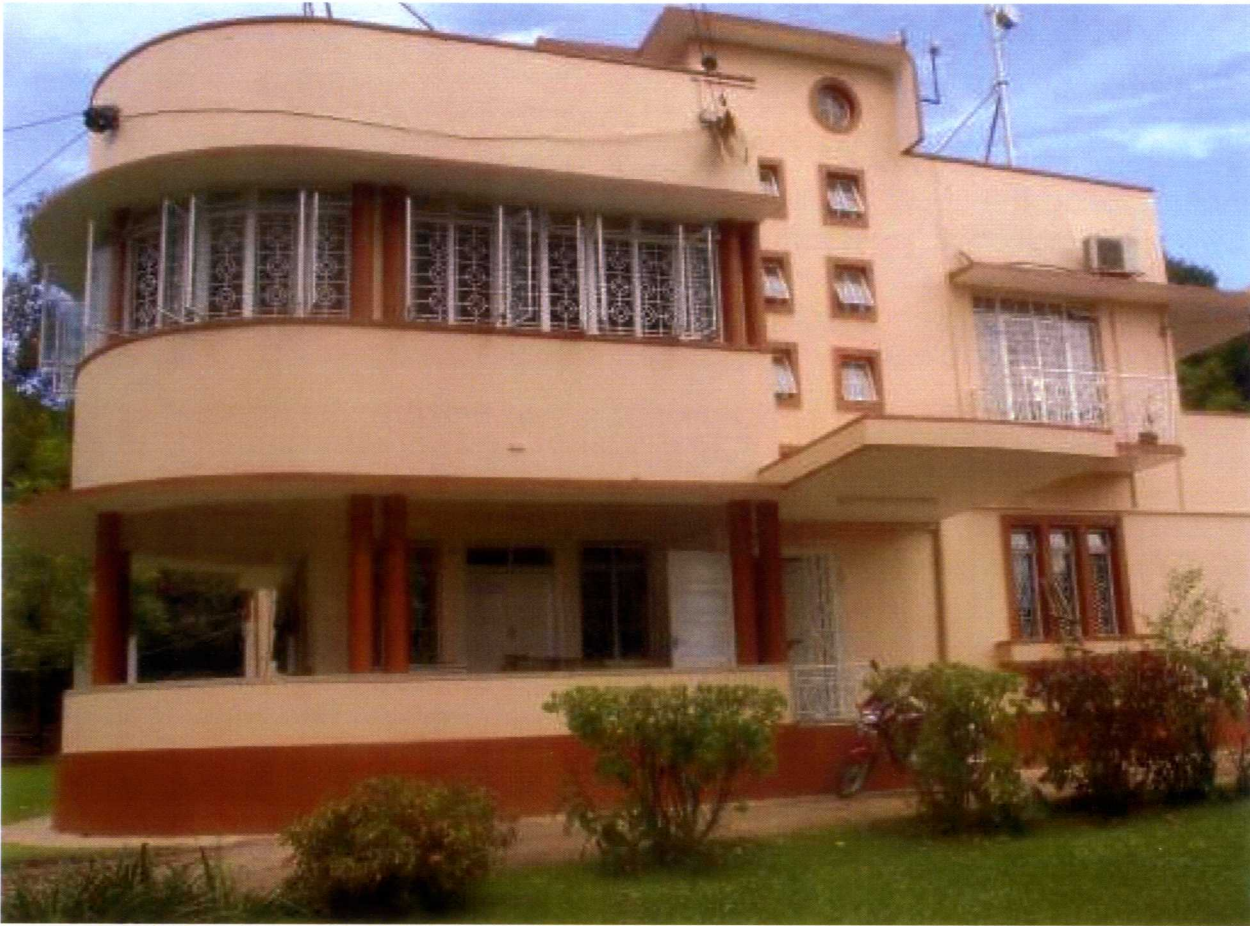
Figure 14: CBR Premises after renovation
