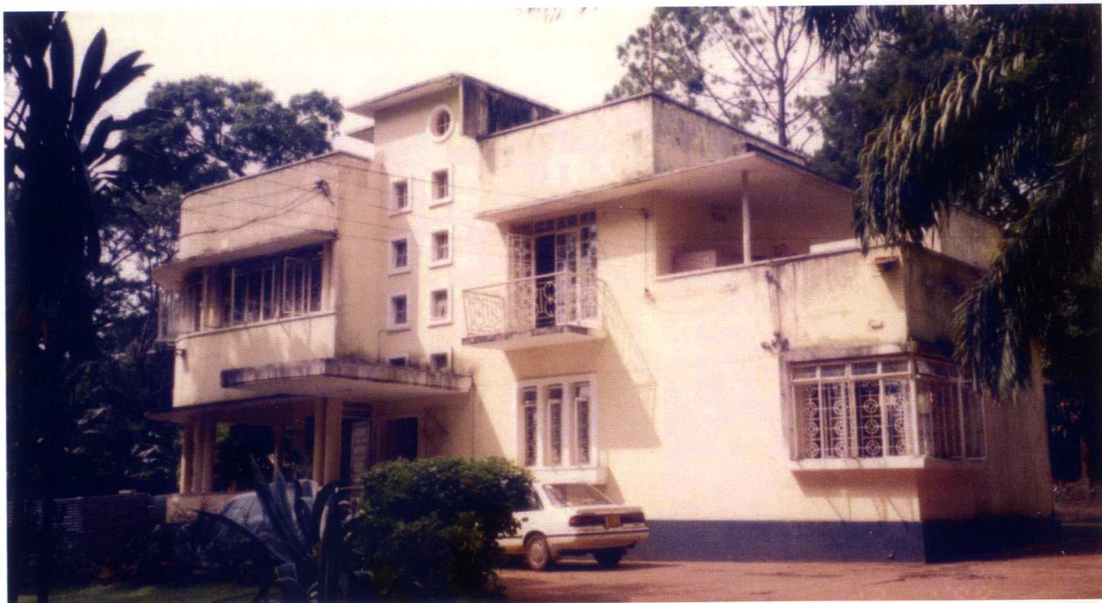
Figure 13: CBR Premises before renovation
